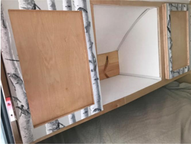
left over from a house project. I chose to only go with a small over head shelf on the front of the cabin and then a large cabinet with 2 doors and an opening for an a/c that will be installed in the future. The interior ceiling is sheets of shelf plastic and then covered with textured wallpaper.
